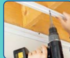
Apply to joists
